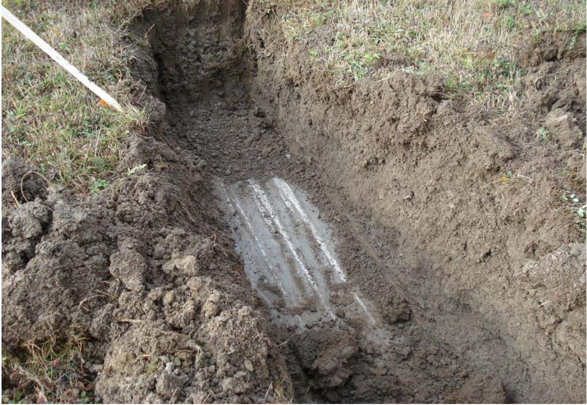
Turbine No. T-50: 50' OS North from Proposed Tower Center
