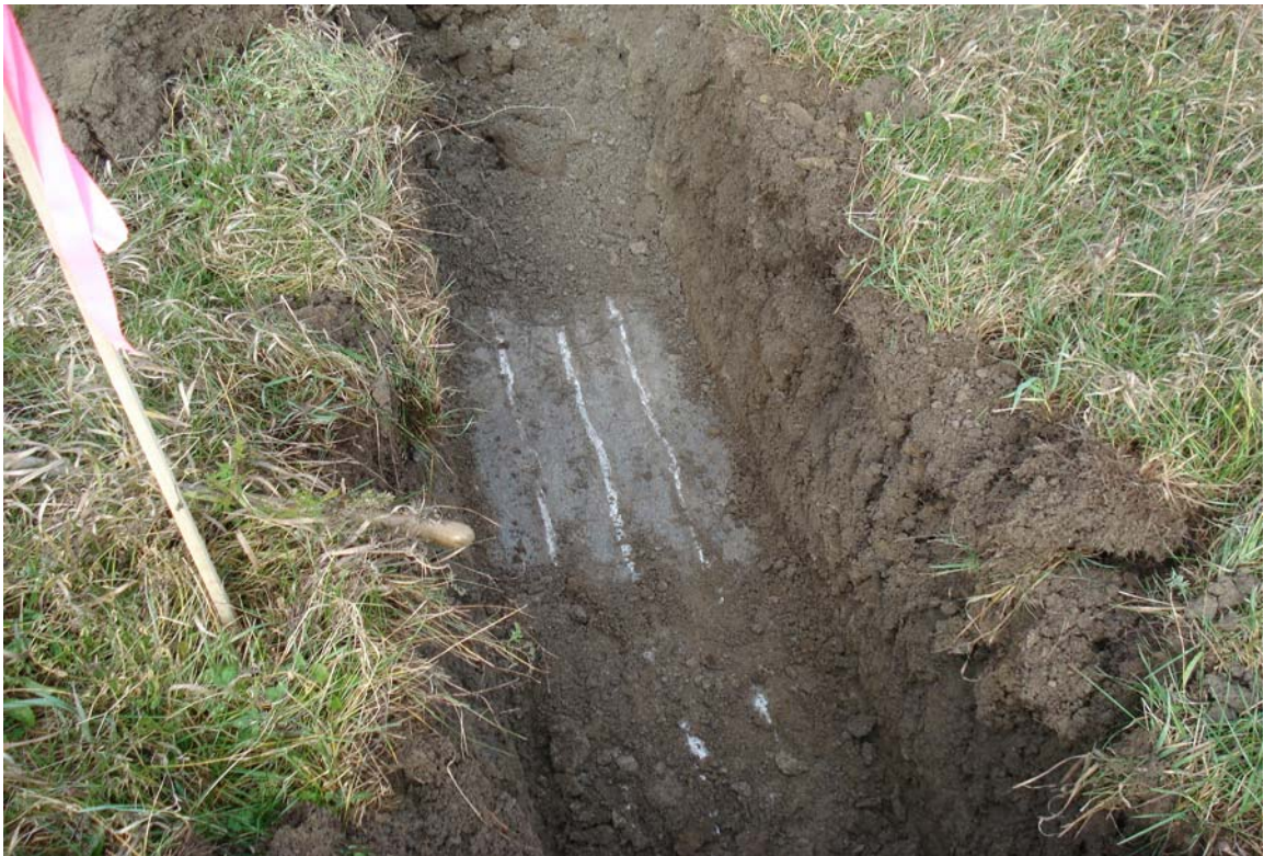
Turbine No. T-20: 50' OS South from Proposed Tower Center
