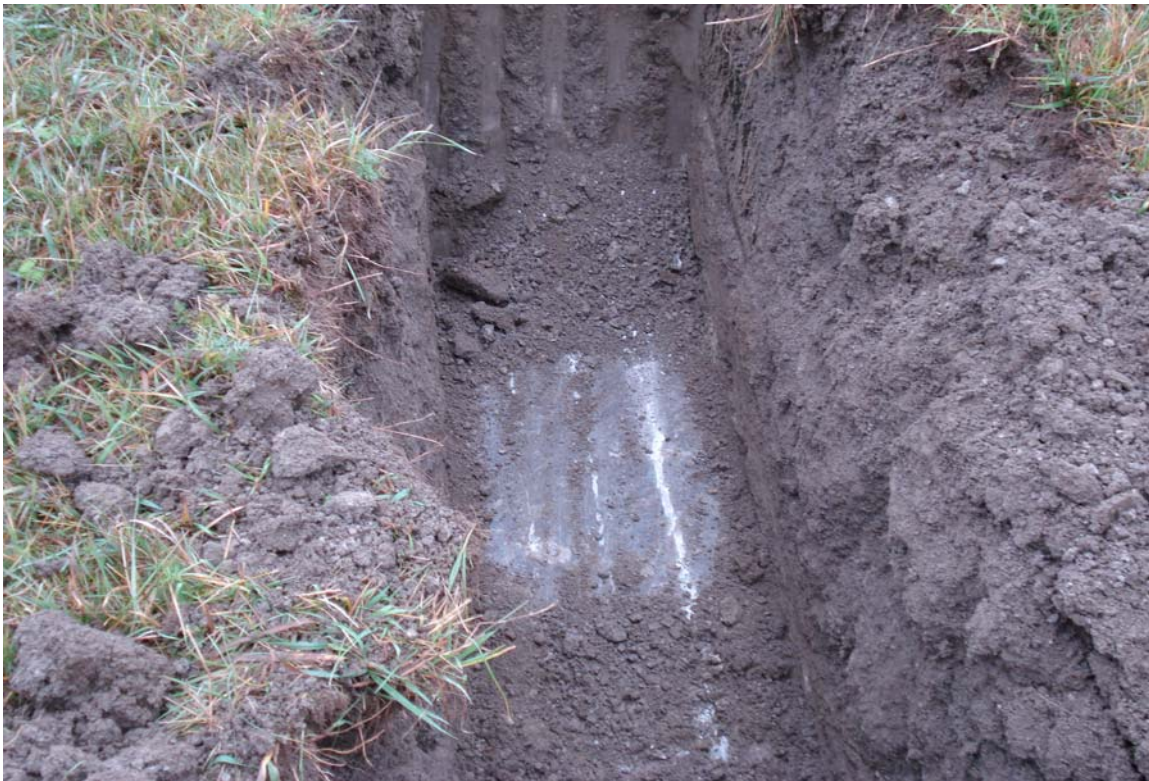
Turbine No. T-42: 50' OS East from Proposed Tower Center
