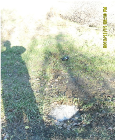
7) Exposed bedrock where significant water flow was heard
