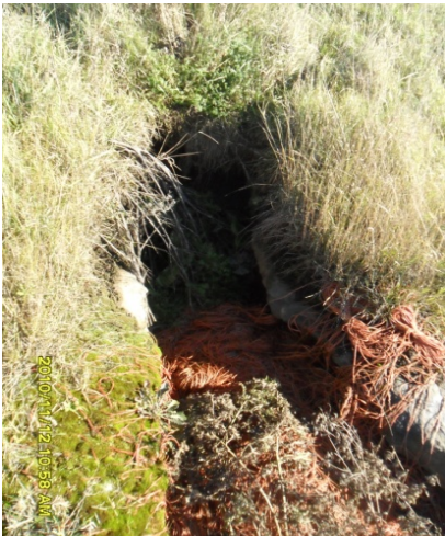
11) Large void and bedrock drain
