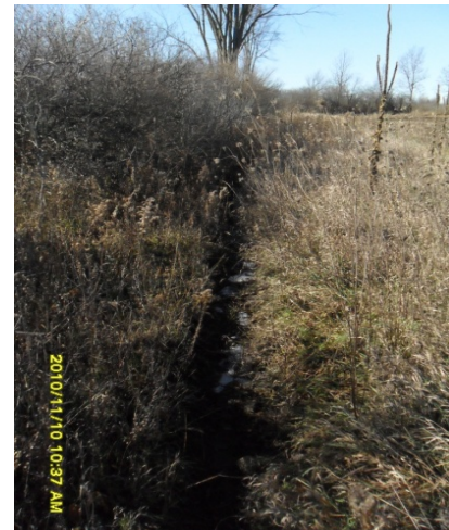
16) Exposed bedrock fracture with voids
