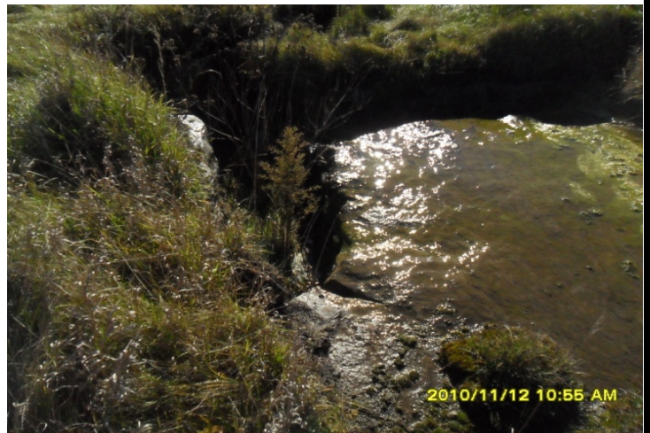
12) Large void and bedrock drain
