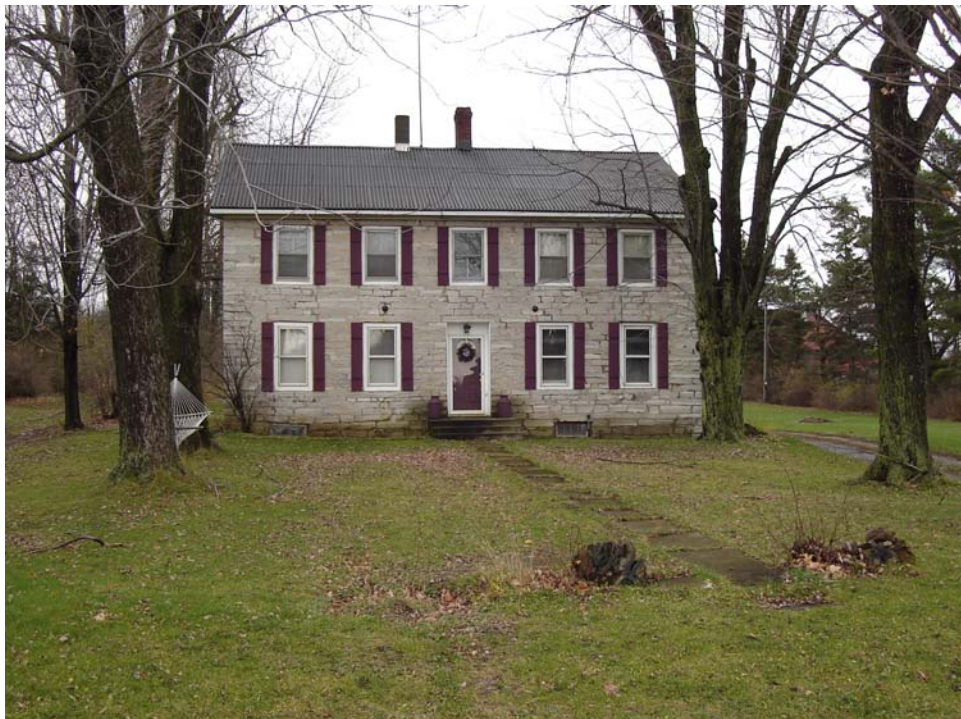
Photograph 4.2. Largely-intact Federal style 5-bay by 2-bay farmhouse with modest quoins (ca. 1820), located at 27192 County Road 54 in the Town of Brownville, Jefferson County ( PCI 2006 ).
