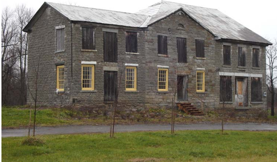
Photograph 4.10. The National Register Listed Irwin Brothers Store (90NR01147) on the northeast corner of NYS Route 180 and Woodward Road, Stone Mills, Town of Orleans (PCI 2006).
