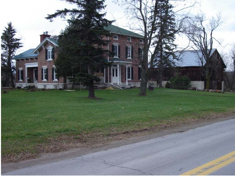
Photograph 4.13. The R. Halladay House in Depauville, Town of Clayton. Constructed in brick, this is a highly-intact example of an Italianate style residence ( PCI 2006 ).
