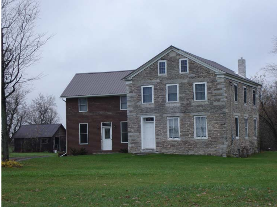
Photograph 4.6. A two-story gable front and wing Greek Revival farmhouse, with a later frame wing. Gable front constructed of local limestone, 1833. Located on Brownville Road in the Town of Brownville (PCI 2006).
