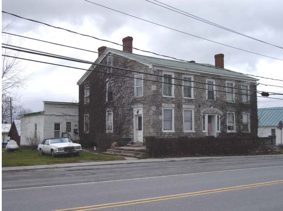
Photograph 4.3. The National Register Listed La Farge Land Office (Orleans Hotel [96NR00962]), NYS 180, La Fargeville, Town of Orleans (PCI 2006)
