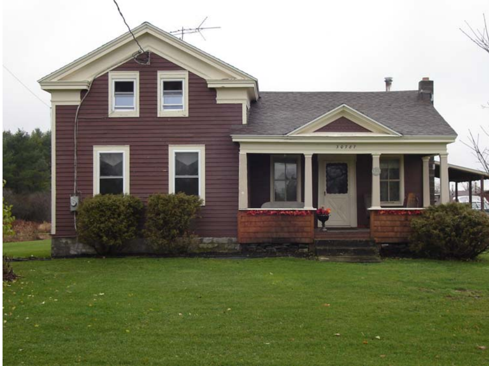
Photograph 4.4. A largely-intact example of a frame, gable front and wing Greek Revival farmhouse, with Craftsman-era porch detail, at 30787 Depauville Road, Town of Brownville. It is in the southwestern portion of the project area ( PCI 2006 ).
