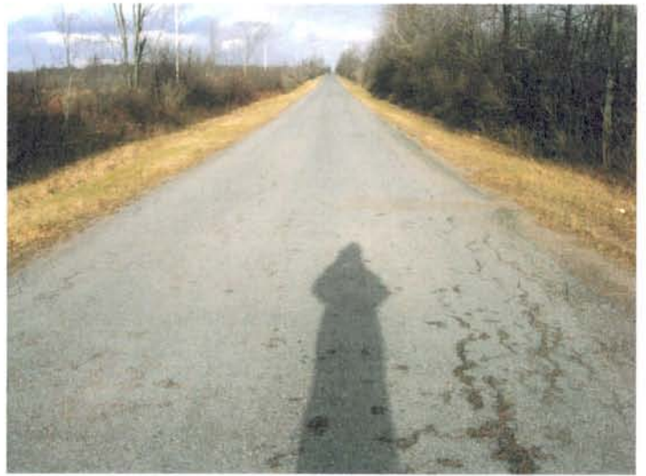
Photograph 20 - Lowe Road east of DePaulville Road
