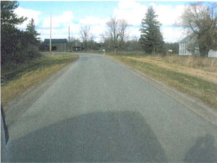
Photograph 9 - Tubolino Road westbound curve
