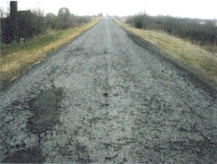
Photograph 21 - Lowe Road west of Sternberg Road
