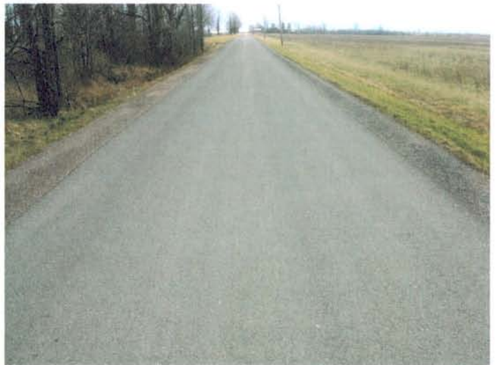
Photograph 4 - Haller Road south of Dutch Gap Road
