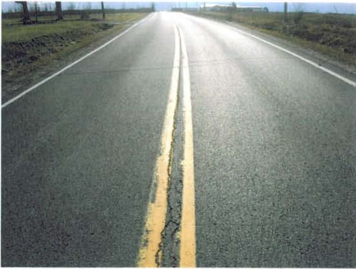
Photograph 1 - NY Route 180 south of County Road 12
