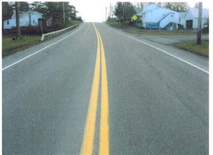
Photograph 30 - NY Route 12 south of County Road 12
