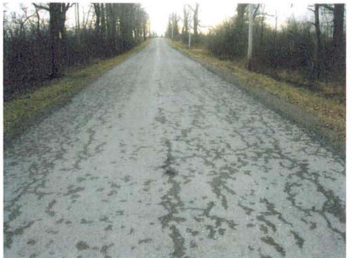
Photograph 24 - Lowe Road west of NY Route 12
