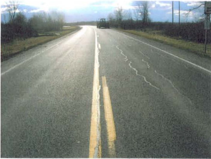
Photograph 13 - NY Route 180 south of County Road 128
