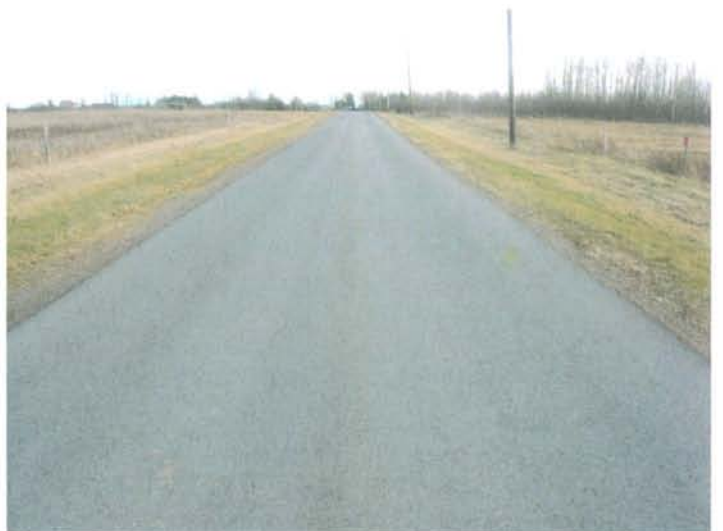
Photograph 6 - Tubolino Road east of Miller Road
